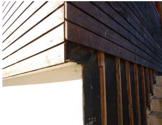
WALL LINING MEMBRANE
