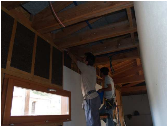
BOARDS BETWEEN STUDS
