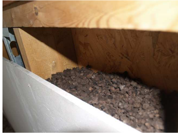
LOOSE FILL GRANULATE BETWEEN STUDS
