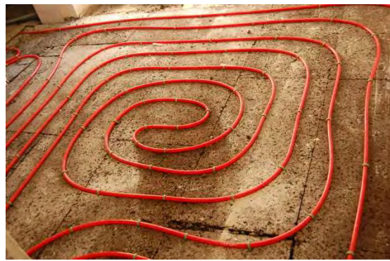
HEATED FLOORING – 1 ST FLOOR
