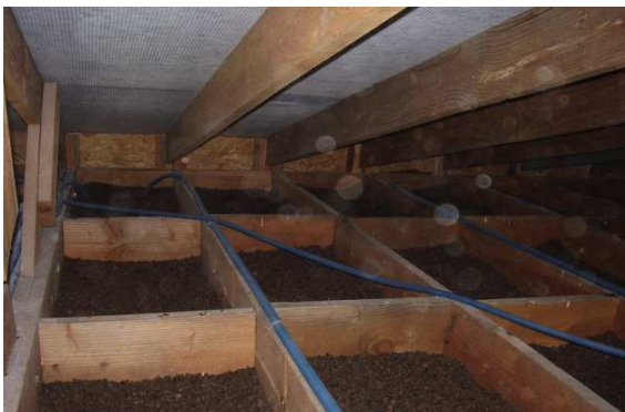
LOOSE FILL INSULATION IN ATTIC
